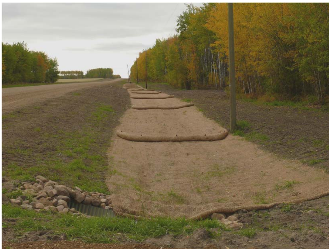
Photo 1. SRFRs installed across the width of a swale.
