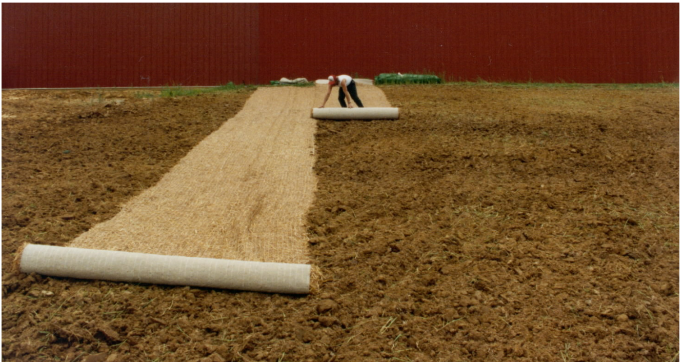
Step Five—Starting at the crest of the slope, roll the RECP down the slope in a controlled manner.
