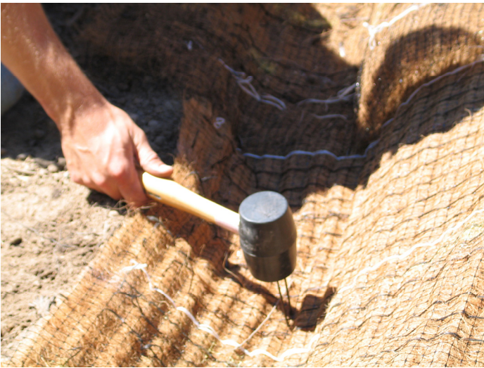
Step Four—Secure the RECP in the anchor trench.
